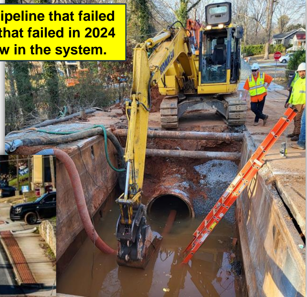
McLendon Road 42" diameter Feb/April 2024 Prestressed Concrete
