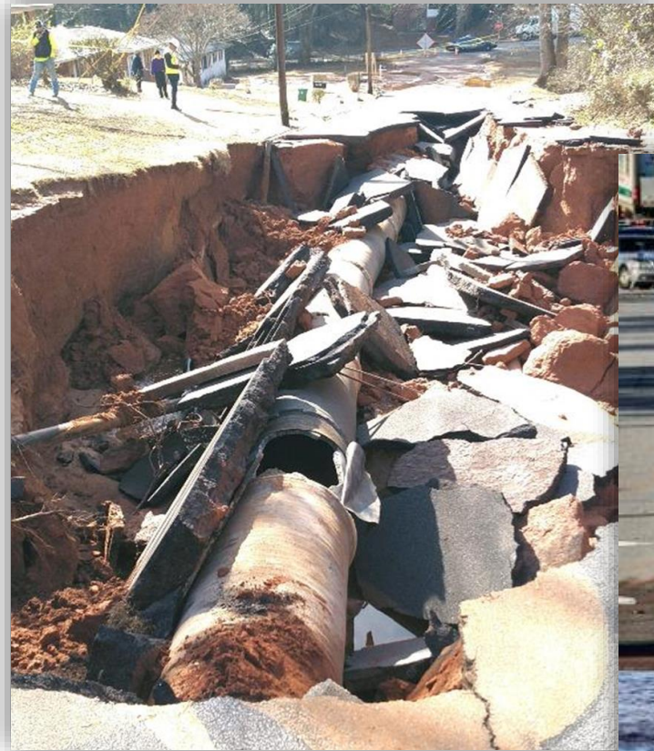
Celia Way January 2023 Prestressed Concrete
